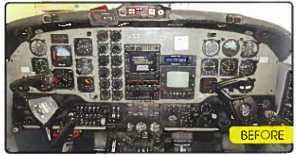
Century Avionics had to remove the complete instrument panel for the installation.
